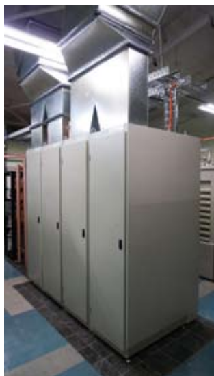
This ETI signal is presented to a highly compact air-cooled Harris solid-state transmitter for broadcasting of the DAB+ RF signal
